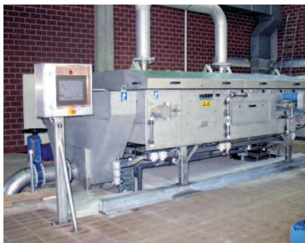
*Drainbelt for up to 100 m<sup>3</sup>/h thin sludge*
